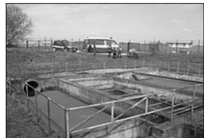
Fig. 3. Lapol D – leaks of oil products.
